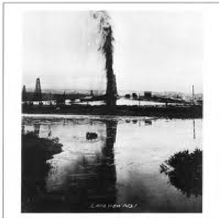
Figure 98—The famous Lakeview gusher that blew in natural seepage in March 1910, Kern, Maricopa and Tarrant Counties. The well flowed for 19 months before it finally quit after producing over 8 million barrels of oil.
